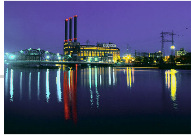
Fig: Power plant.
