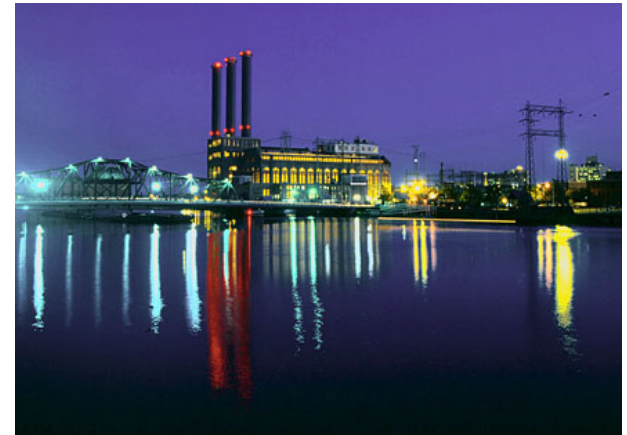
Fig: Power plant.
